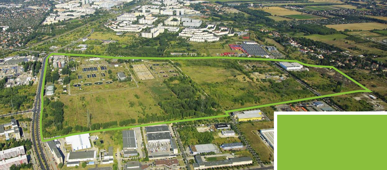
Area plan for the upcoming Clean Tech Business Park Berlin-Marzahn (Photo: Stefan Otto – Aperçu Verlagsgesellschaft)
